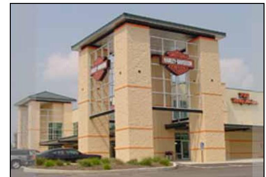
BES was responsible for site layout, utilities extension and design to meet a very rigorous schedule.
